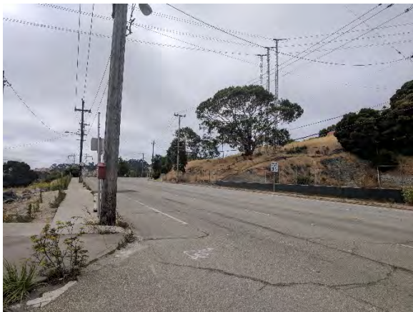
Figure 5. Hunters Point Boulevard, viewed facing southeast from Evans Avenue
