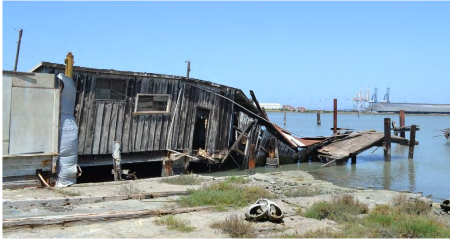
Figure 41. Southeast façade, viewed facing north
