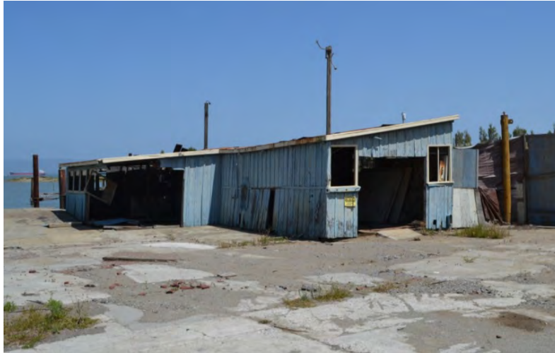
Figure 37. Southwest façade of the blacksmith and machine shop, viewed facing east
