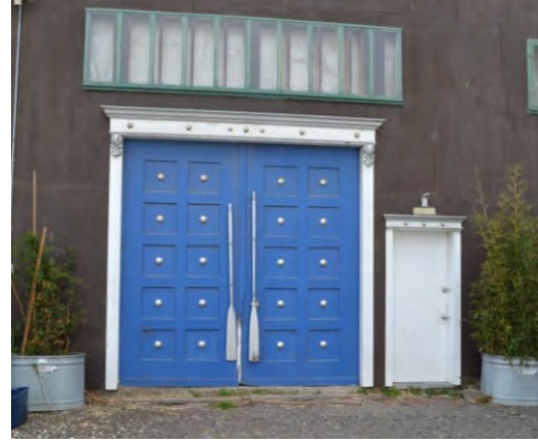
Figure 19. First-story doors, viewed facing southwest
