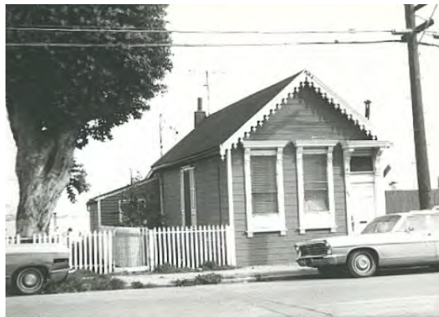
Figure 116. Shipwright’s cottage, as photographed by the Planning Department in 1976; the bathroom addition near the west corner of the house had not yet been built.
