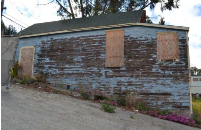
Figure 8. Northeast façade, viewed facing south
