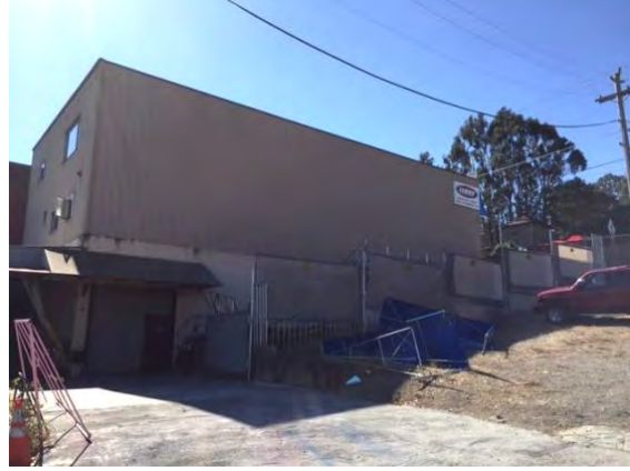
Figure 85. Northwest façade, viewed facing southeast Source: Build Inc.
