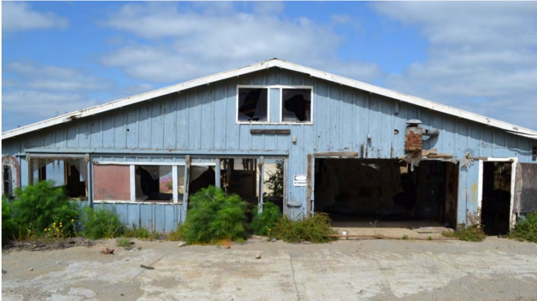
Figure 45. Southwest façade, viewed facing northeast
