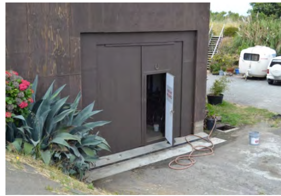
Figure 24. First-story entrance located at the east end of the façade
