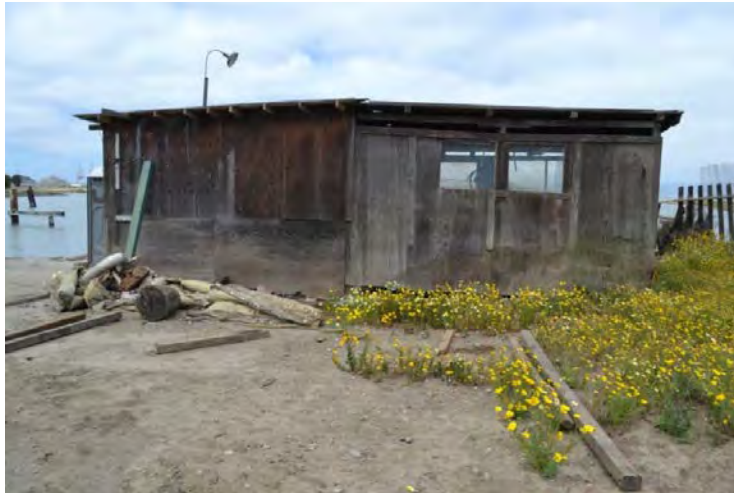
Figure 73. Southwest façade of the storage building, viewed facing northeast
