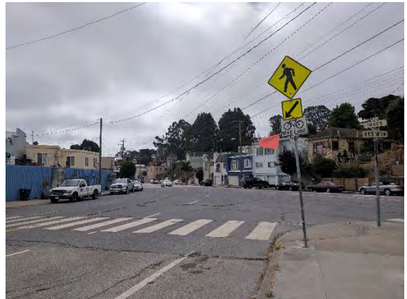
Figure 10. Intersection of Hunters Point Boulevard and Innes Avenue, viewed facing southeast
