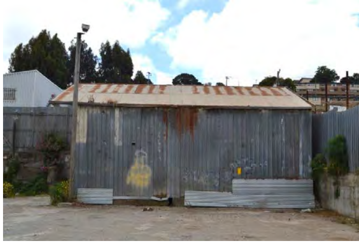
Figure 57. Northeast façade, viewed facing southwest
