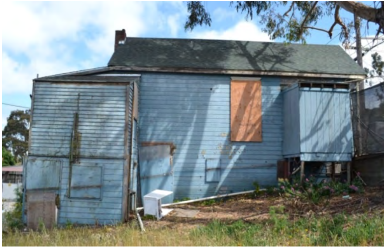
Figure 12. Southwest façade, viewed facing northeast
