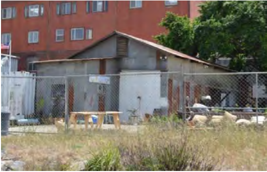
Figure 77. Northeast façade, viewed facing south
