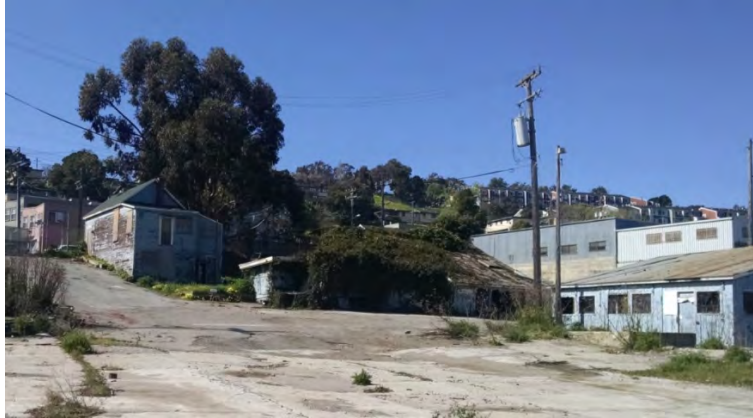
Figure 34. Buildings belonging to the India Basin Scow Schooner Boatyard site, viewed facing southwest
