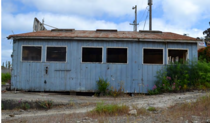
Figure 47. Northwest façade, viewed facing southeast
