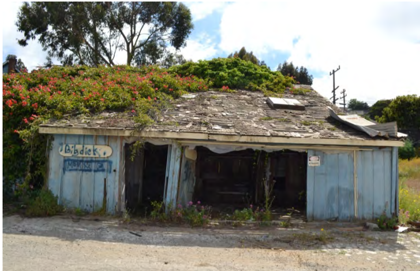
Figure 52. Front (northeast) façade of the tool shed (at left, obscured by vegetation) and water tank house, viewed facing southwest
