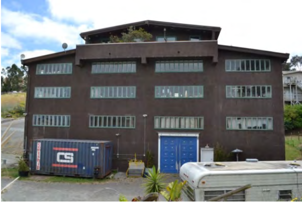
Figure 18. Northeast (primary) façade, viewed facing southwest
