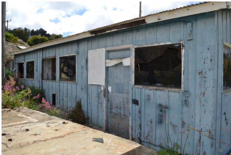
Figure 44. Southeast façade, viewed facing west
