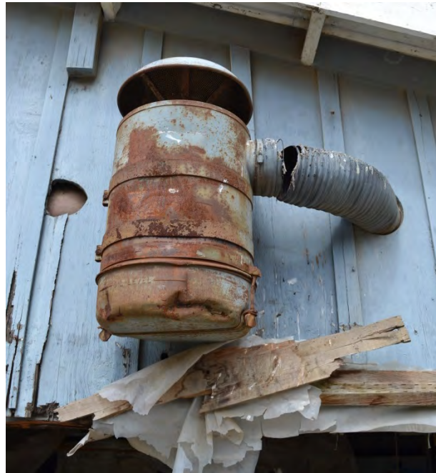
Figure 46. Detail of mounted ventilator
