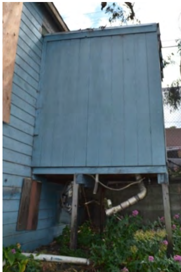
Figure 13. Projecting bathroom addition at northwest façade, viewed facing southeast
