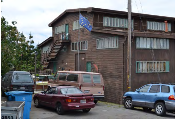
Figure 21. Southwest façade, viewed facing north
