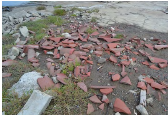
Figure 67. Broken concrete and terra cotta fragments located at the central construction way
