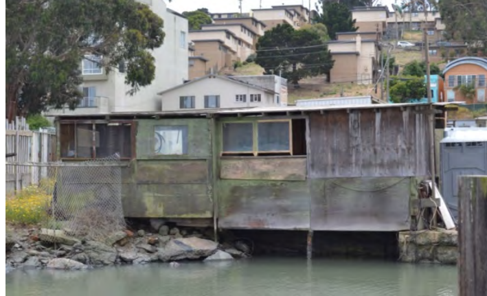
Figure 75. Northeast façade, viewed facing southwest
