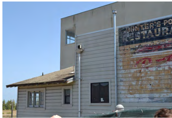
Figure 30. Northwest façade, viewed facing east
