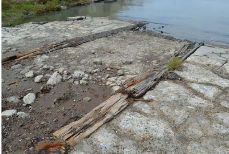
Figure 35. Embedded marine way track and concrete ramp of west marine way
