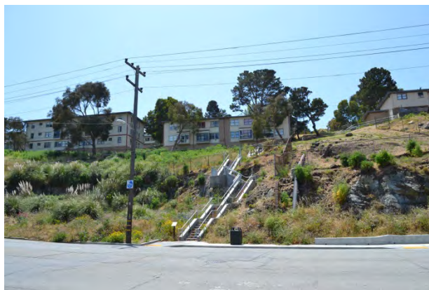
Figure 98. Former public housing buildings at the Hunters Point ridge, viewed from Innes Avenue at its intersection with Arelious Walker Drive
