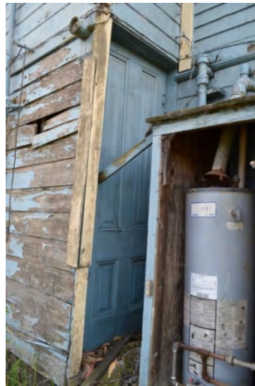
Figure 14. Molded panel basement door at north corner of the northwest façade, viewed facing east
