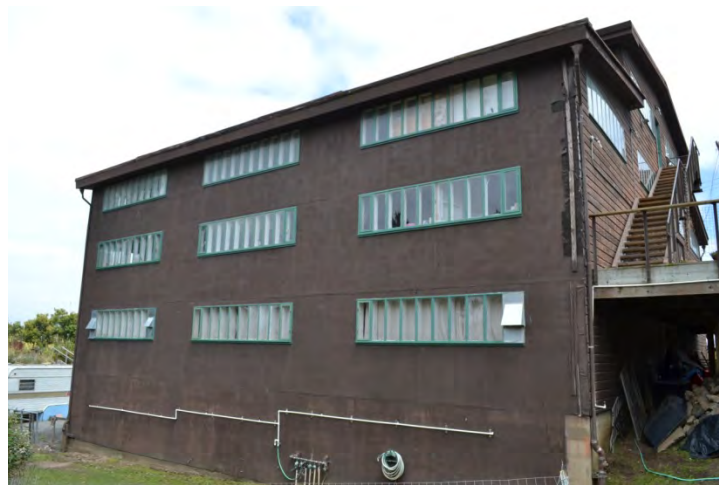
Figure 20. Northwest façade, viewed facing east
