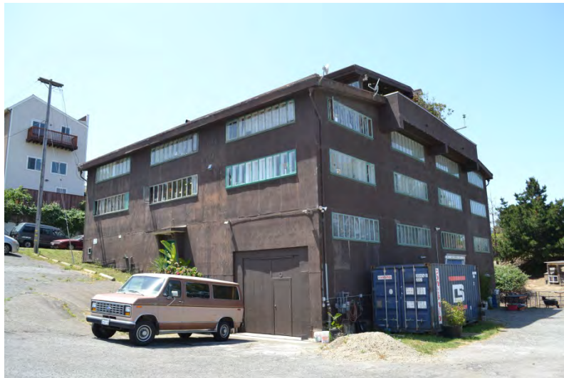
Figure 17. Oblique view of northeast and northwest façades, viewed facing south
