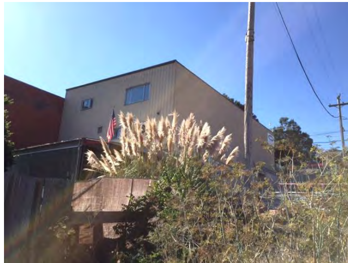
Figure 86. Rear façade, viewed facing south Source: Build Inc.
