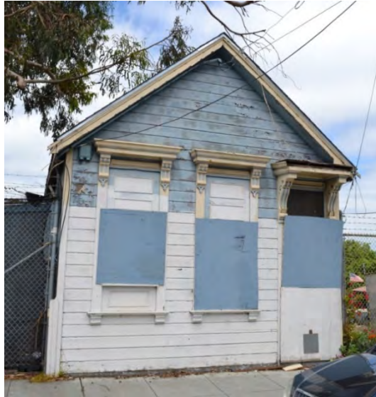
Figure 5. Primary (southeast) façade, viewed facing northwest
