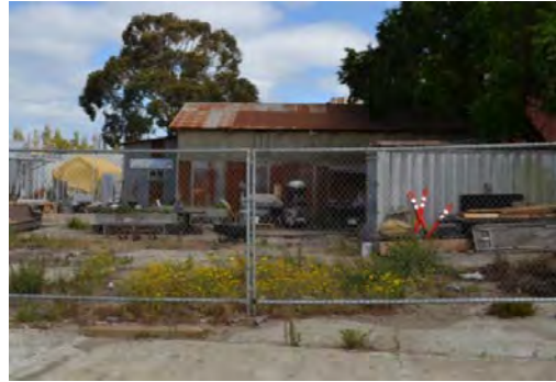
Figure 78. Northwest façade, viewed facing southeast
