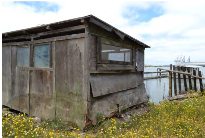
Figure 76. Southeast façade, viewed facing north
