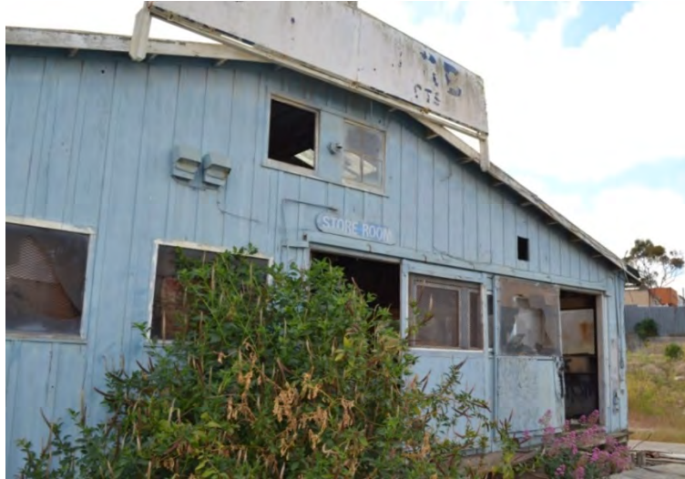
Figure 43. Primary (northeast) façade, viewed facing west
