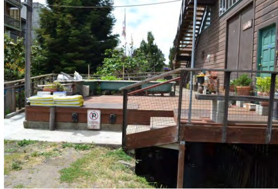
Figure 22. Wood deck, viewed facing northwest
