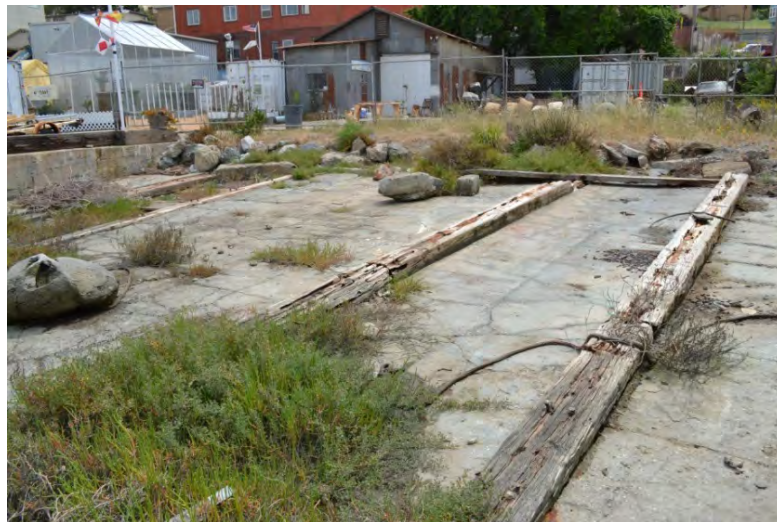
Figure 36. Marine ways and concrete ramp of the east marine ways
