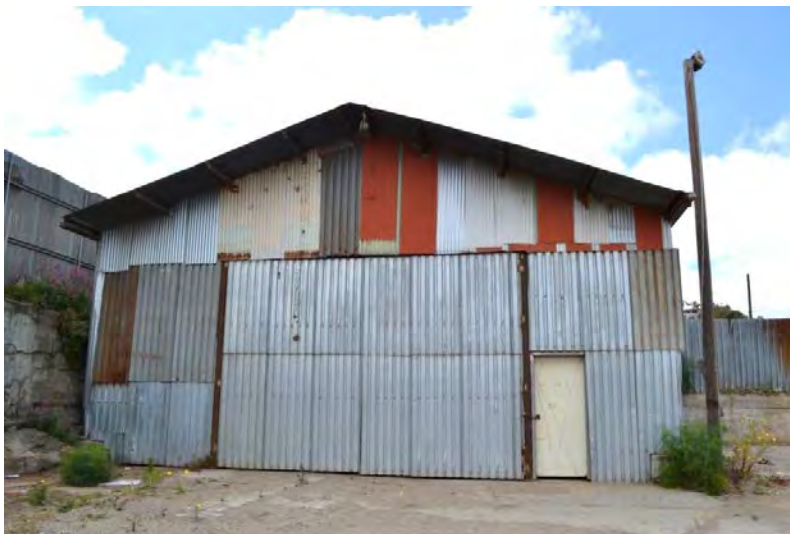
Figure 56. Front (southeast) façade, viewed facing northwest
