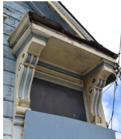
Figure 7. Door hood and bracket detail
