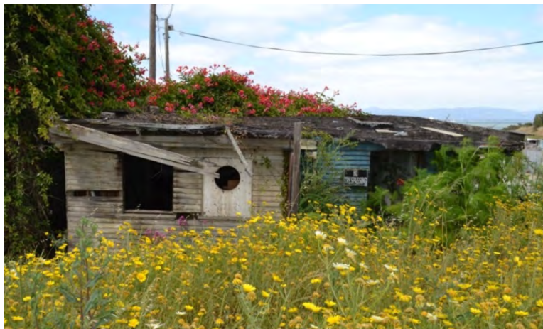
Figure 50. Southwest façade, viewed facing northeast
