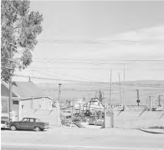
Figure 134. The Anderson & Cristofani Boatyard, viewed from Innes Avenue through the main entrance, 1964; the Shipwright's Cottage is at left Source: Maritime Research Center, San Francisco Maritime National Historical Park
