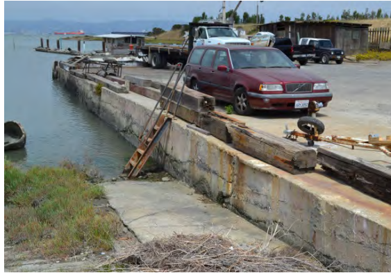
Figure 71. Northwest edge of the Allemand Brothers wharf, alongside the east marine ways of the India Basin Scow Schooner Boatyard, viewed facing northeast
