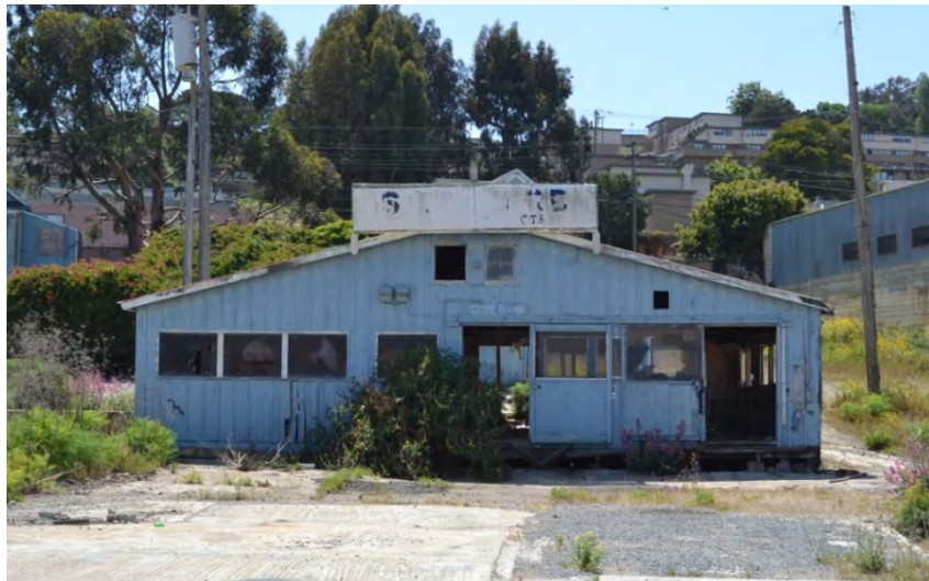
Figure 42. Front (northeast) façade of the paint shop and compressor house, viewed facing southwest
