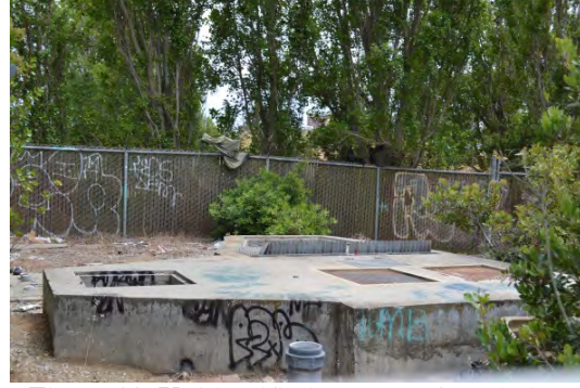
Figure 92. Unidentified concrete foundation within fenced area
