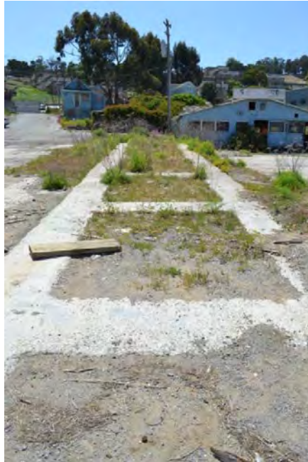
Figure 61. Central construction way foundation, viewed facing southwest from the boatyard wharf towards the compressor house and paint shop, and the Shipwright's Cottage beyond
