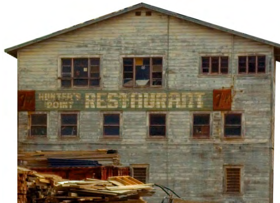
Figure 127. Undated photograph of the building's rear façade Source: flickr user kristineenea
