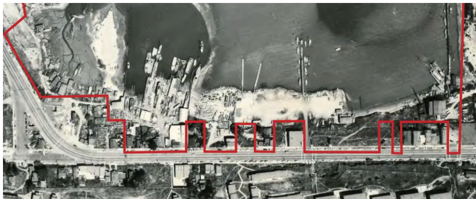
Figure 109. This 1958 aerial photograph shows that infilling had begun at either end of India Basin, with the current project boundary marked; upper left is north. Source: Pacific Aerial Surveys, edited by Page & Turnbull
