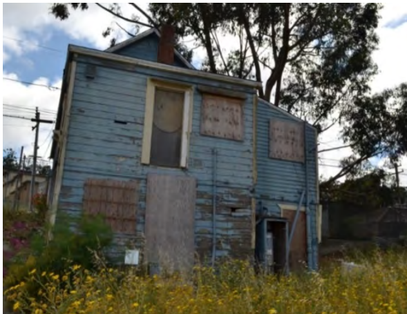
Figure 10. Northwest façade, viewed facing southeast
