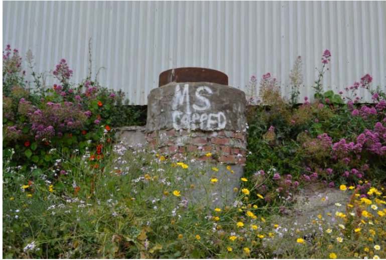
Figure 65. Sewer standpipe, viewed facing northwest
