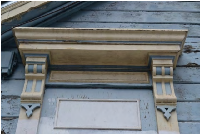
Figure 6. Window transom panel and architrave detail
