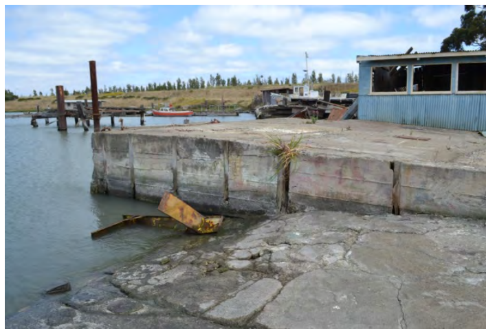
Figure 58. Southeastern half of the concrete wharf, raised above the central construction way ramp, viewed facing east
