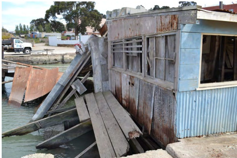
Figure 40. Rear (northeastern) façade, much of it collapsed, viewed facing south
