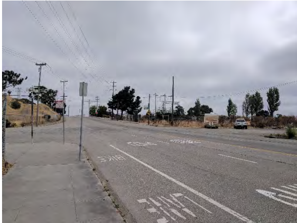
Figure 7. Intersection of Hawes Avenue and Hunters Point Boulevard, viewed facing north
