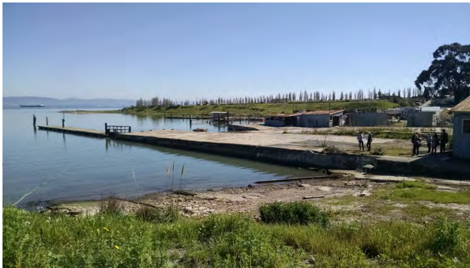
Figure 33. India Basin inlet, viewed facing southeast
