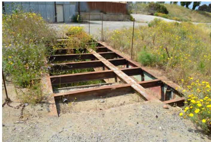
Figure 62. Exposed steel road undergirding, viewed facing northwest
