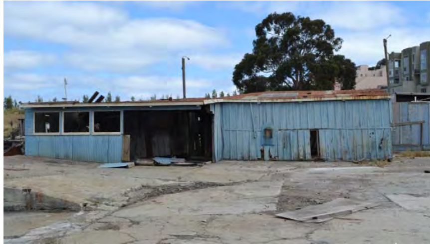
Figure 39. Northwest façade, viewed facing east
