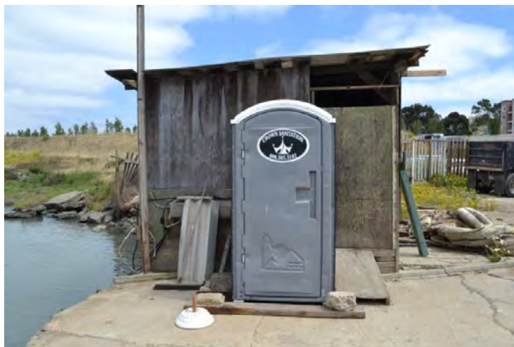
Figure 74. Northwest façade, viewed facing southeast
