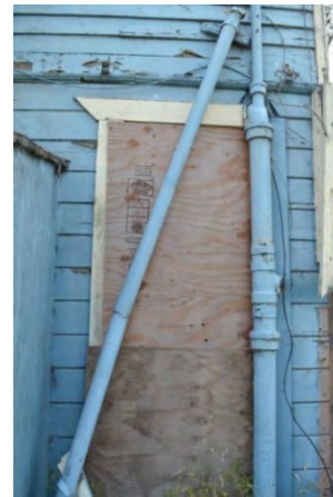
Figure 11. Boarded basement door opening at northwest wing
