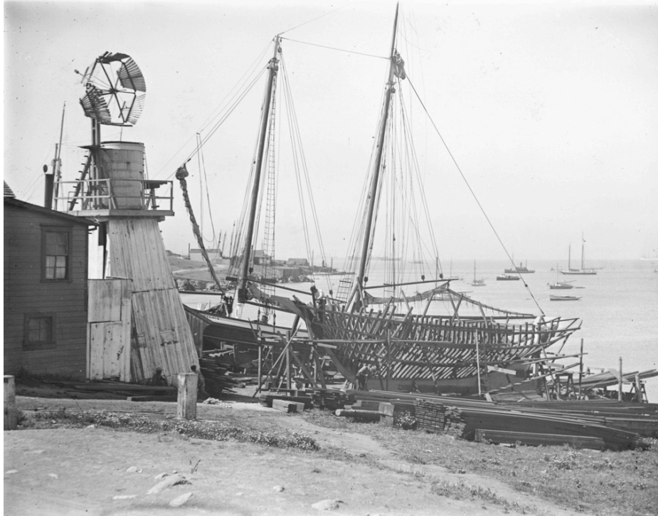
Figure 128. Jack London's boat, the Snark , under construction at Pop Anderson's yard, 1907. The rear wing of the Shipwright's Cottage and the attached well and windmill structure are visible at left, indicating the shoreline of India Basin lay noticeably closer to the residence than it does currently.
