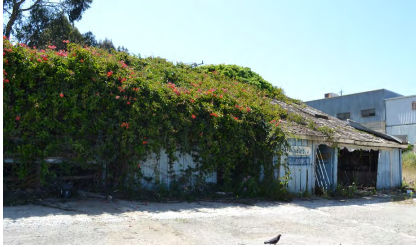
Figure 51. Oblique view of the tool shed and water tank house, viewed facing west
