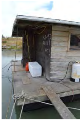
Figure 81. Northeast façade, viewed facing south
