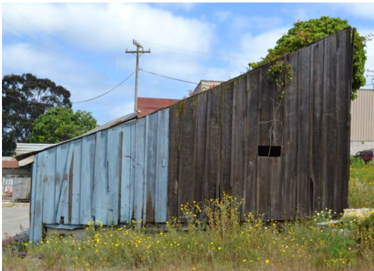
Figure 54. Northwest façade, viewed facing southeast
