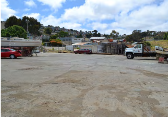
Figure 70. Wharf of the Allemand Brothers Boatyard, viewed facing west towards the neighboring India Basin Scow Schooner Boatyard
