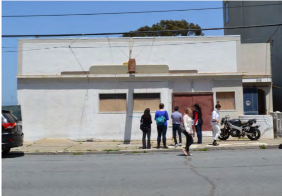
Figure 27. Southwest (primary) façade, viewed facing northeast
