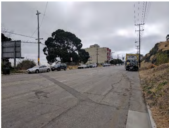
Figure 17. Innes Avenue viewed facing southeast from Arelious Walker Drive
