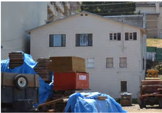
Figure 29. Northeast (rear) façade, viewed facing southwest
